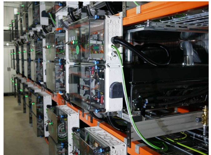
Fig. 20. Interior view of the second-life LSS in Lünen (source: GETEC Group).
